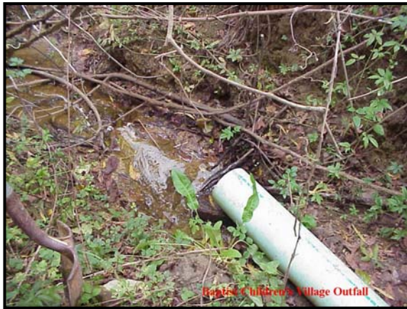
Photo 3.1. Outfall for Baptist Children's Village
